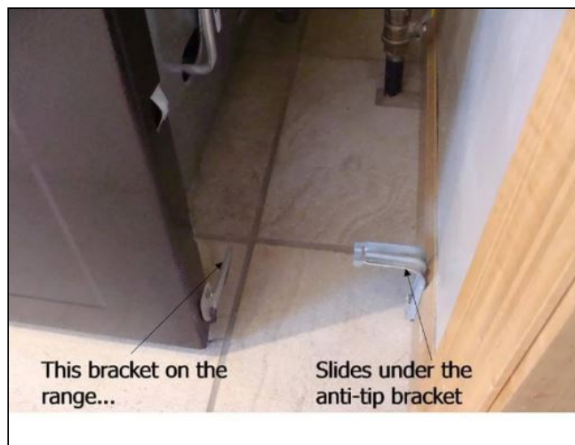
11.2 Item 3 (Picture) Anti Tilt Bracket Diagram Photo
