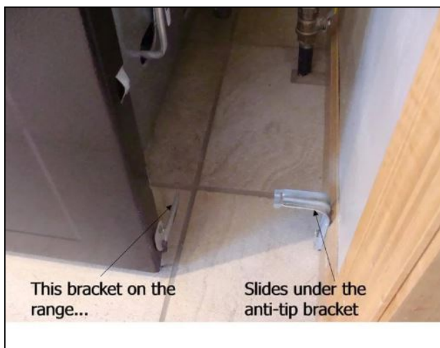
11.2 Item 3 (Picture) Anti Tilt Bracket Diagram Photo
